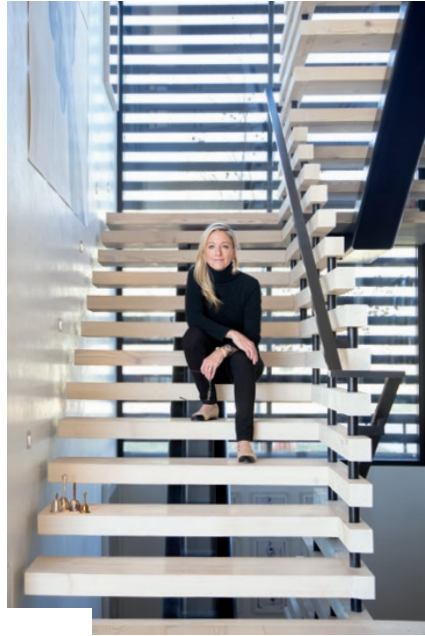
Alexa Wesner on her home’s central stairwell, an Escher-like functional sculpture with open risers and treads that also serve as handrails
